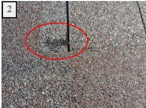
Apparent mechanical damage in several locations
