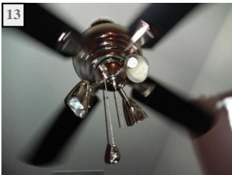
In upstairs den. Two lamps are missing, one appears to be burned out.
